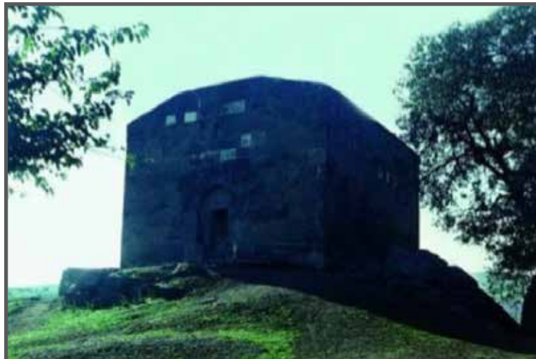
Garghabazar mosque in Fuzuli built in 1681. Was destroyed after the occupation of Fuzuli in 1993. 72
